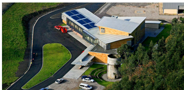
Aerial view of the Tunnel Fire and Ventilation Research Centre, San Pedro de Anes. Fundación Barredo.
