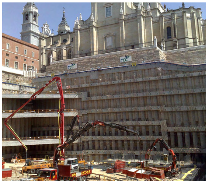
Construction of phase one, Museum of Royal Collections
