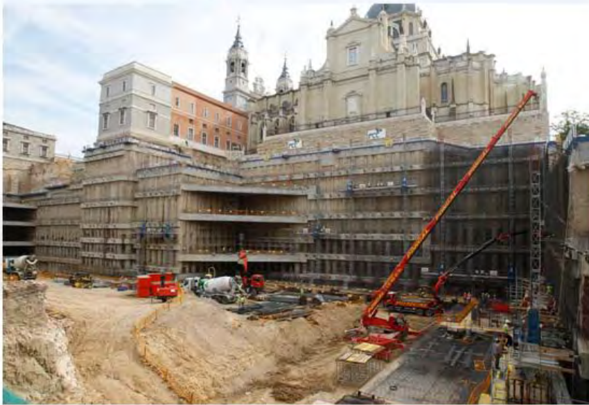
Retaining wall for the Museum of Royal Collections. Plaza de la Armería. Madrid.
