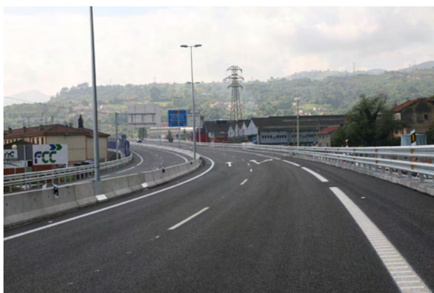
Autovía de los Túneles dual carriageway, section between Riaño and Sama
